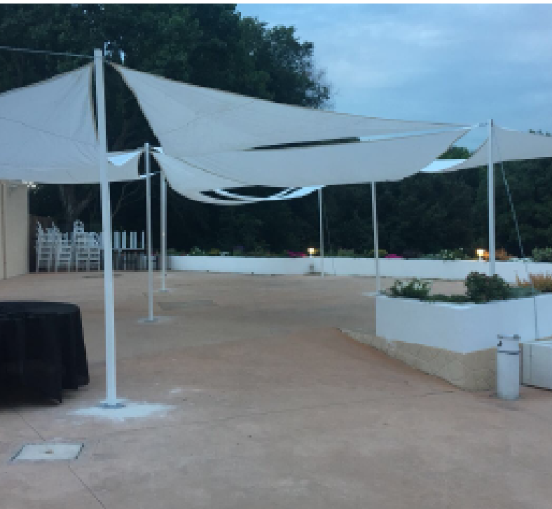
Example of installation with Maanta sails, NOT correctly tensioned and tilted, and NON-Maanta poles.
